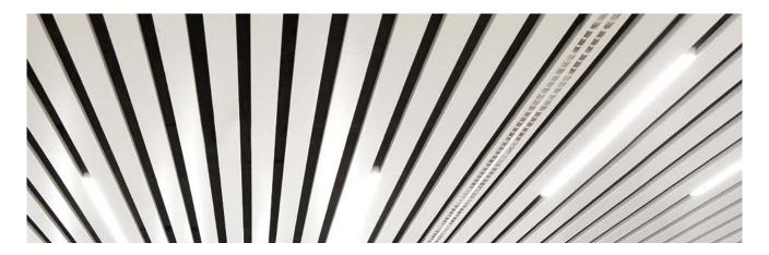
SAS720 is a 'plank' system, available in a variety of widths and depths depending on aesthetic preference. Highly robust and sturdy, SAS720 is suitable for service integration as an integral design feature, offering significant creative flexibility.
