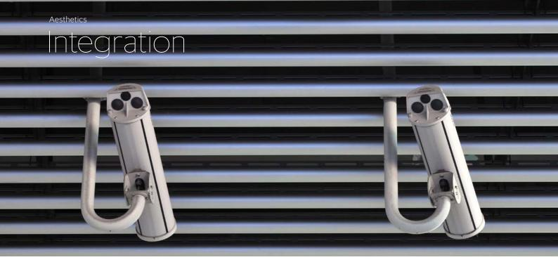
One of the most significant design benefits of metal is the ability to fully integrate M&E services within the ceiling. This can be anything from lighting and speakers to sprinkler systems. Detailing is controlled in an aesthetically pleasing manner, integral to the overall design concept. Apertures can be pre-formed during manufacturing to ensure the installation mirrors the design intent.
