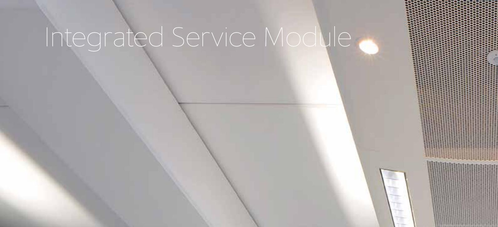
SAS ISMs aesthetically encase an active or passive chilled beam within an architectural metal casing. Sometimes referred to as Multi-service Chilled Beams (MSCB), ISMs integrate most building services such as lights, sensors and smoke detectors.
