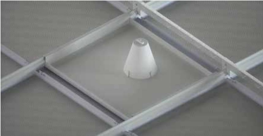
Lighting and other services can be integrated with SAS150. Modular lighting can be supported directly from the soffit. Where maximum point loads are exceeded (2.5Kg) the service must be supported independently or from the grid.
